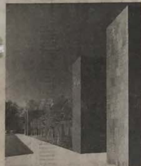
The usual procedure for a new post office is to go to a drawer and pick out a blueprint specified for the city's size and needs, to exactly resemble all the others. Miller persuaded the government to let him supply original plans. Roche and Dinkeloo did the honors.
