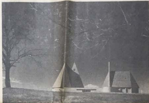
The Athens of the Prairie is strong on churches. This one, with echoes of antiquity in modernism, was designed by the Chicago firm of Harry Weese. It wraps around a center courtyard.
