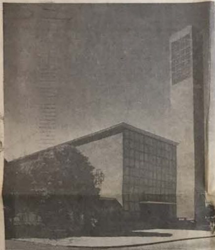
Elia Saareinen's First Christian Church, 1942, set the precedent for topflight architecture to follow. Note asymmetrical accents of the structure, inspired by a traditional Italian church with bell tower.
