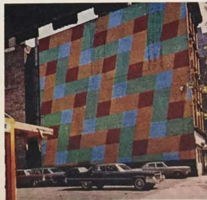
Colorful, slanted checkerboard overlooks parking lot. Building, to come down soon, is at 17th St. and Third Ave.
