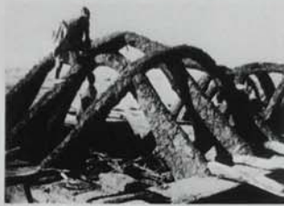
153 Method of vault construction at Talawa, Nigeria.
