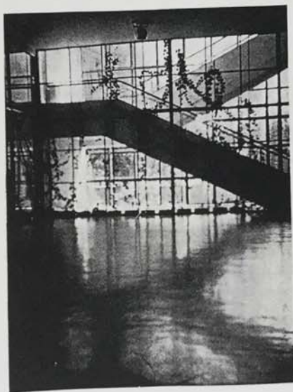
12 Library, Viipuri, 1934. Interior view of main staircase. The metal window divisions form a trellis for the vines which are planted in boxes along the landings.
