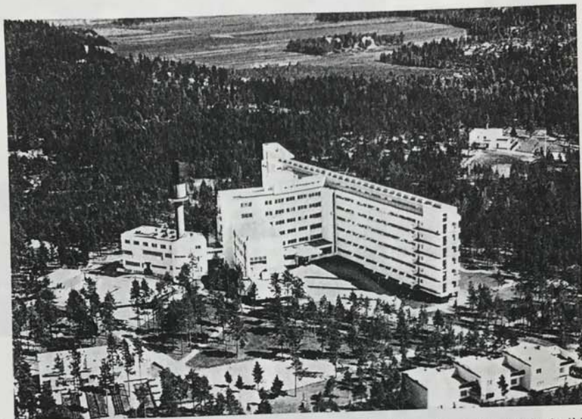
2 Tuberculosis Sanatorium, Paimio, 1932. Air view of site. The various wings of the building are oriented for maximum light and air.
