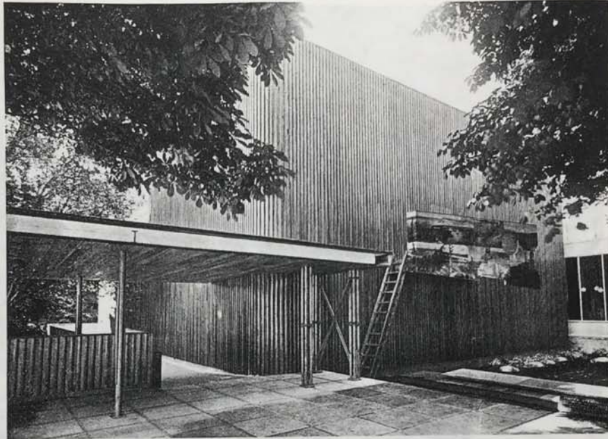
18 Finnish Pavilion, Paris, 1937. North elevation and open loggia showing vertical ribbed boarding with which building is faced and mushroom-like lights in garden.
