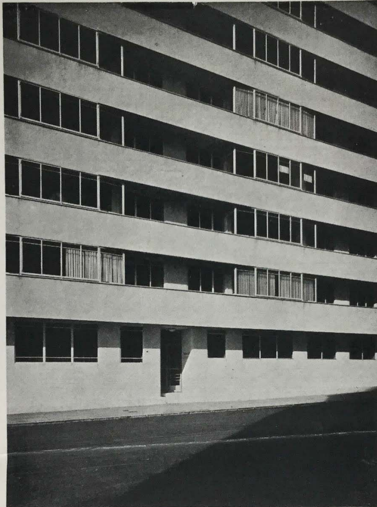
A detail of the side elevation showing typical balconies and windows
