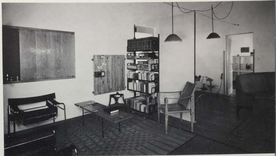
Above: Chessa has equipped his living room for maximum flexibility. Bar and china cabinets built into wall (latter projecting) can be reached from dining room side of wall. Partition is one of two that slide on track. Bookcase is mobile too.
