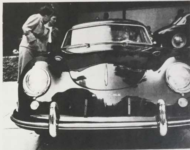
"LID ON A TRAY" design, here exemplified by the German Porsche, a rich man's offshoot from the much touted Volkswagen. The engine is in the rear.
