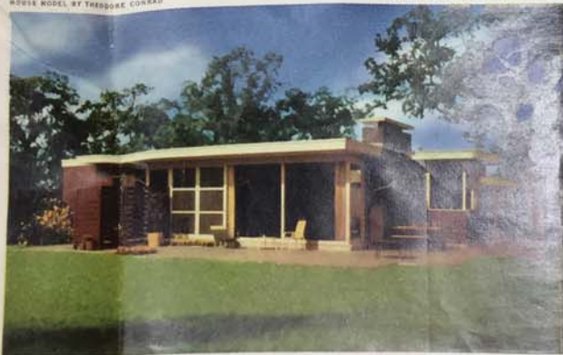
Garden side: This side is largely a combination of clear and obscure glass. The obscure glass, plus a section of fence, affords privacy to the parents' bedroom at extreme left.
