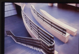
Atrium railing, concrete and painted steel
