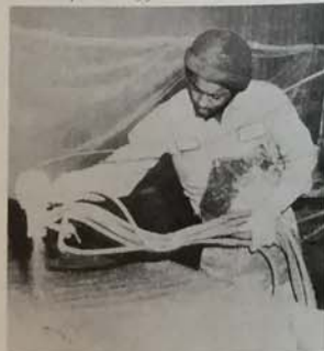
GFRC is sprayed into its formwork.
