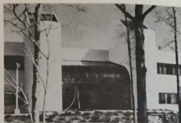
The ITT Office Complex, Shelton, Ct (GSGS & D), shown here makes use of spray-applied GFRC for the curved panels and factory cast-in-place flat panels.
