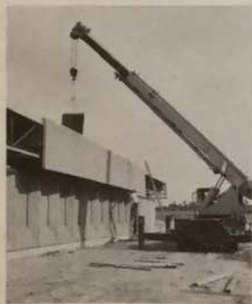
The economy of FRC panels results from ease of handling, transportation and erection allowed by the lightweight material.
