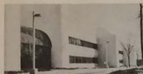
The ITT Office Complex, Shelton, Ct (GSGS & D), shown here makes use of spray-applied GFRC for the curved panels and factory cast-in-place flat panels.
