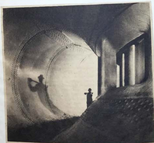
The 1930s—The magic of the age of steel and concrete, harnessing the forces of nature for man's benefit and better living—a dramatically effective shot at the scroll case of a hydraulic generator in the Tennessee Valley Authority's power plant, by Charles Krutch, TVA official photographer.
