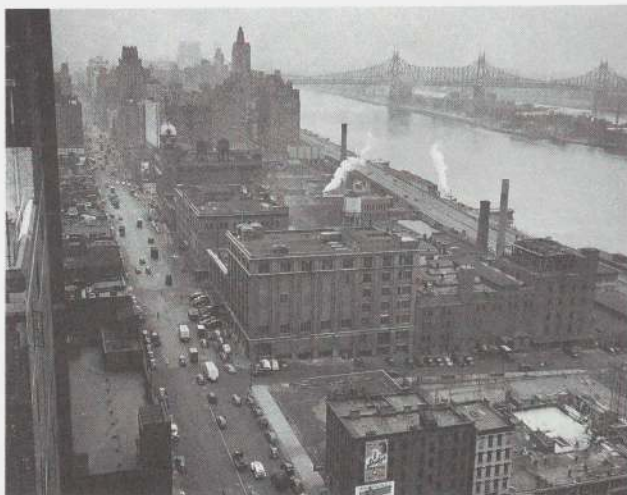
3. Site of the United Nations Headquarters, New York, looking north from 41st Street. December 12, 1946. Photo: United Nations
