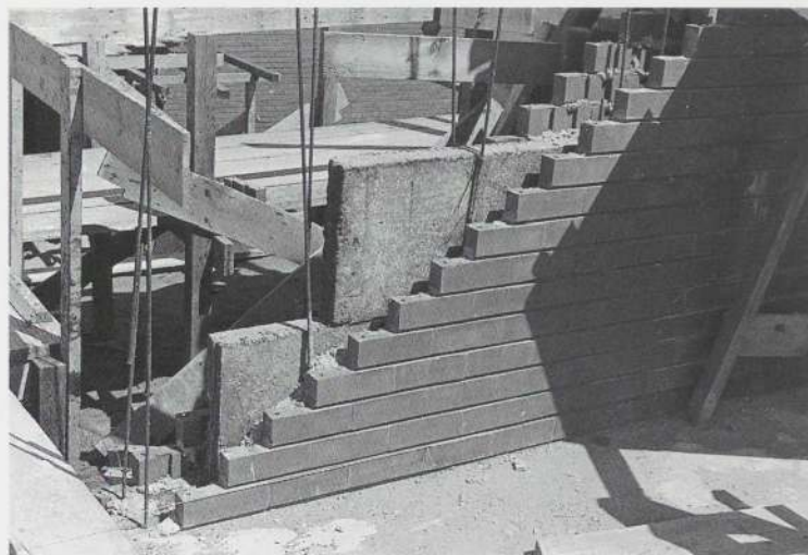
Figure 19: Frank Lloyd Wright. S. C. Johnson & Son, Inc. Administration Building, Racine. 1936–39. Exterior wall under construction
