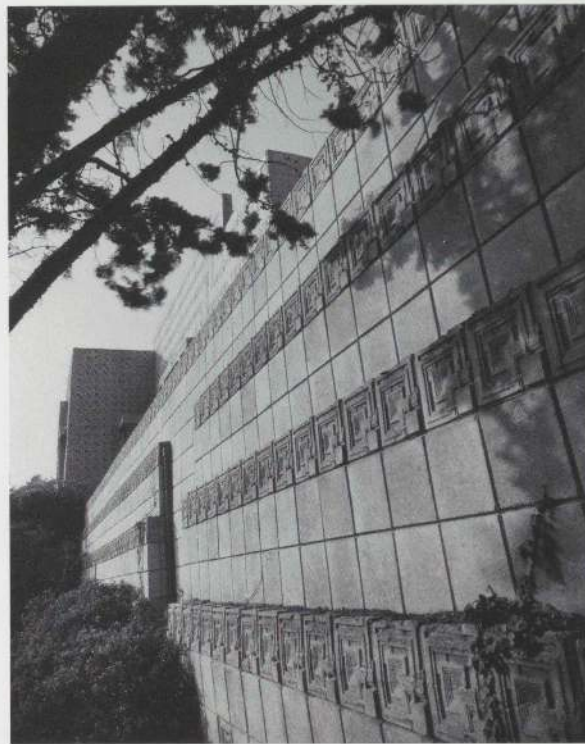
Figure 5: Frank Lloyd Wright. Exterior detail, Charles E. Ennis House, Los Angeles. 1923–24
