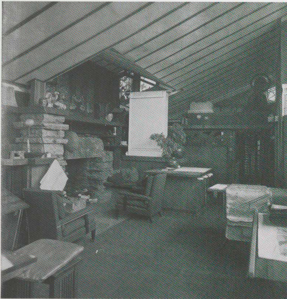
Taliesin II FRANK LLOYD WRIGHT HOUSE AND STUDIO Spring Green, Wisconsin, 1914 (partially destroyed)
