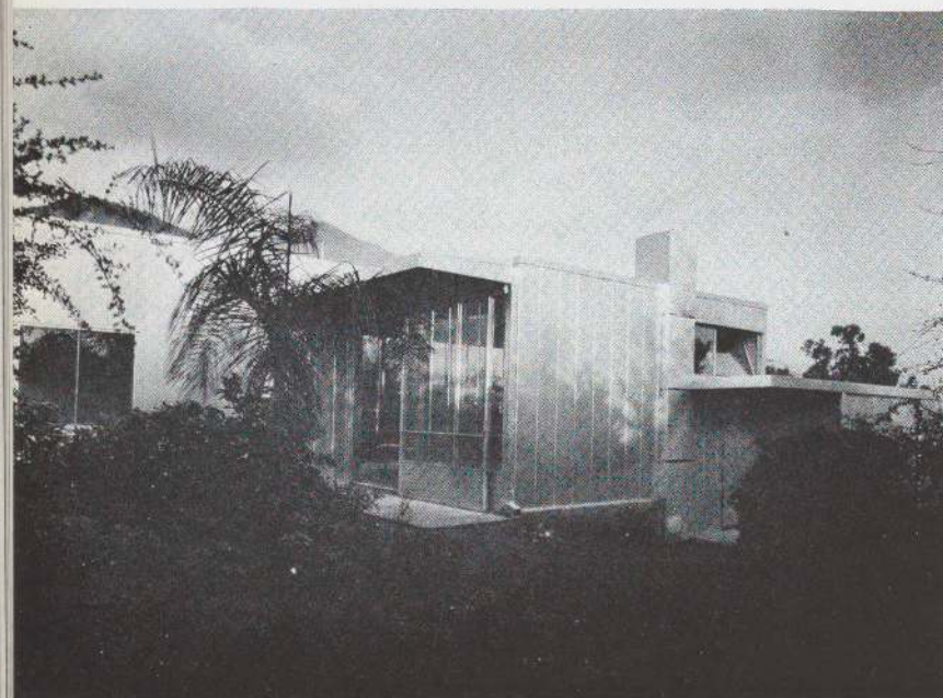
House assembled of narrow pre-fabricated panels of insulated steel. (Richard J. Neutra: house in Altadena, Cal.)
