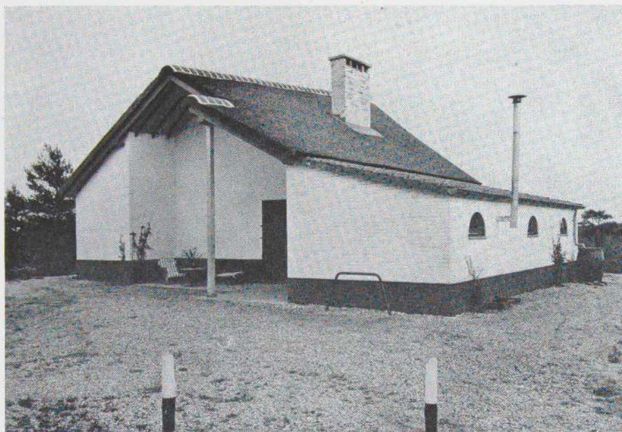
The Dutch have always had a way with brick. Notice the massive walls and forthright arched window openings of this recent house by a well-known modern Dutch architect. (G. Rietveld: house in Tongeren, Holland.)
