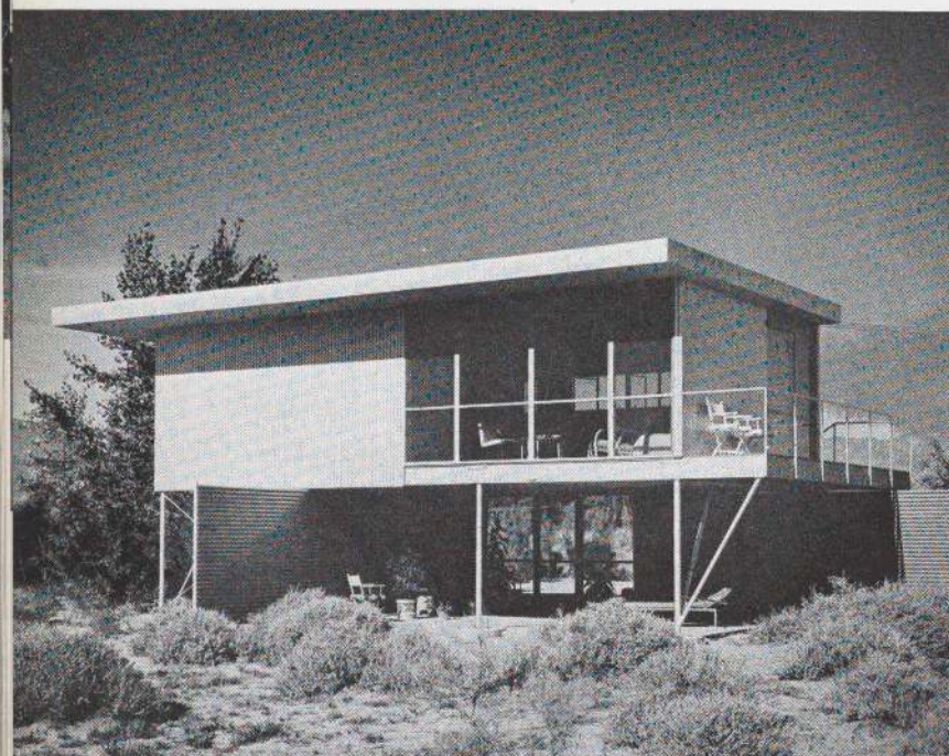
Steel pipes lift the body of the house from the ground. Walls are of standard wood studs with an exterior facing of corrugated iron. (John Porter Clark and Albert Frey: vacation house in Palm Springs, Cal.)
