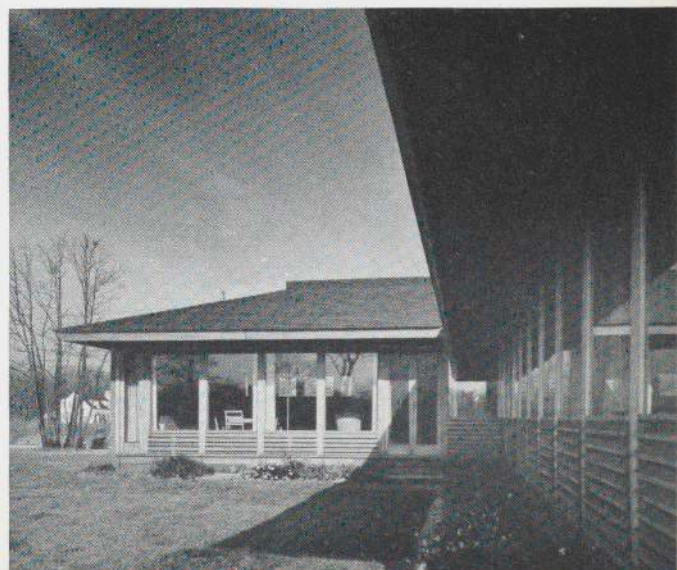
In both of the houses shown below, air circulates through slatted transoms set below or above immovable panes of glass. (Left. George Fred Keck: prefabricated "Solar" house. Right. Paul Schweikher: house in Glenview, Ill.)
