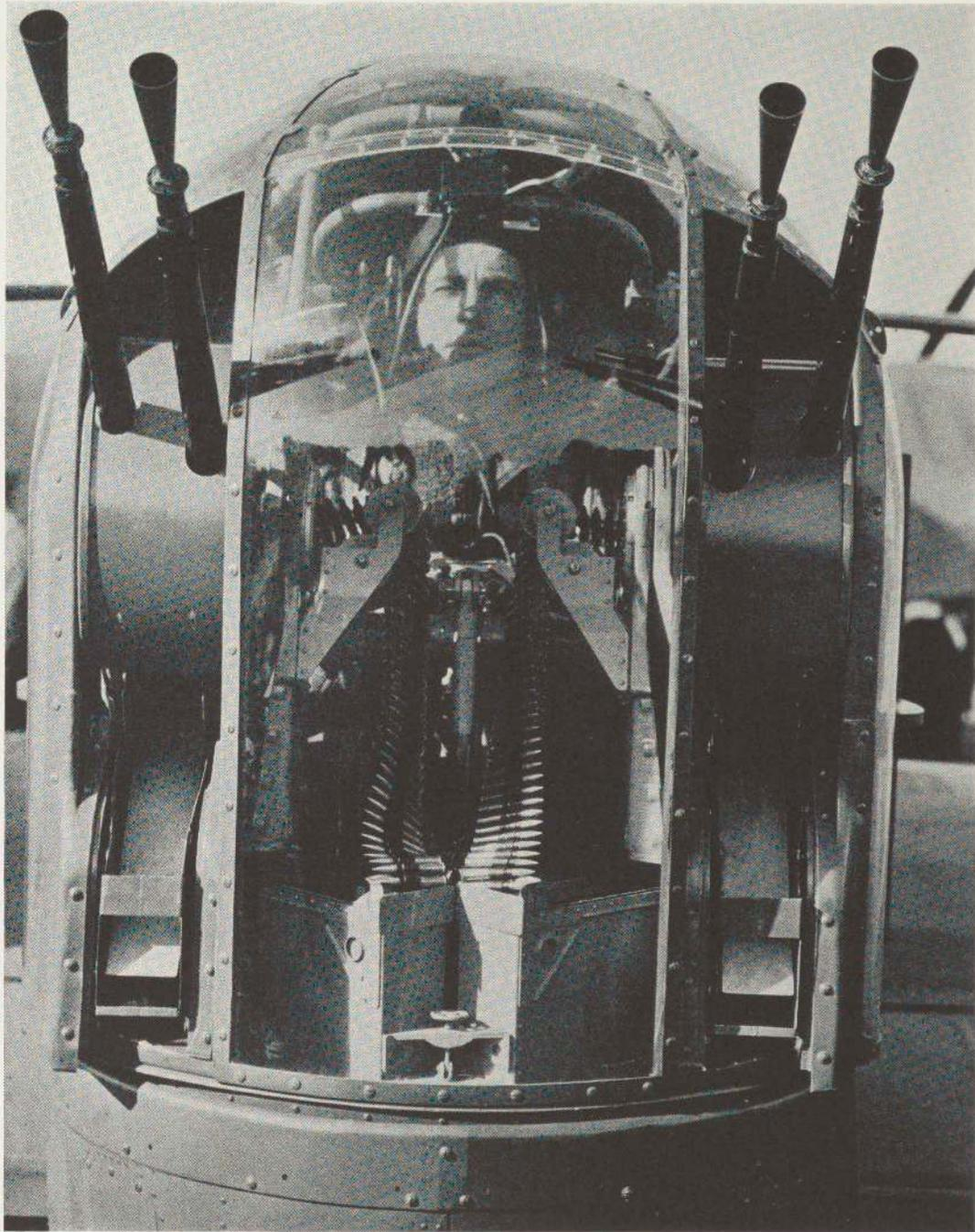
*REAR TURRET OF A WHITLEY BOMBER. At the top may be seen four Browning machine guns, with flash eliminators, capable of firing 4,800 shots a minute. In the center bullets may be seen above the ammunition boxes. The chutes on either side discharge empty cartridge cases. The gunner is in a highly vulnerable position. His is a night vigil, and often he must maintain his watch for ten hours at a time.*
