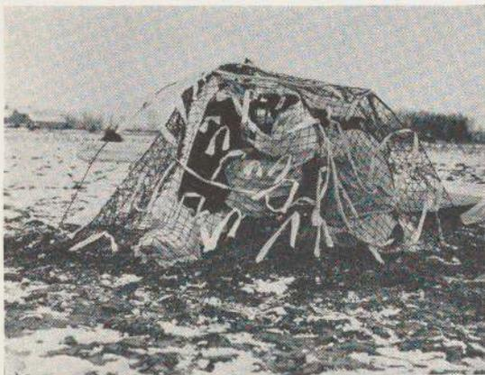
AN ANTI-TANK GUN concealed with fishnet. The gunners are wearing white. A few strips of white cloth tied into the netting imitate the sparse pattern of snow on the ground.
