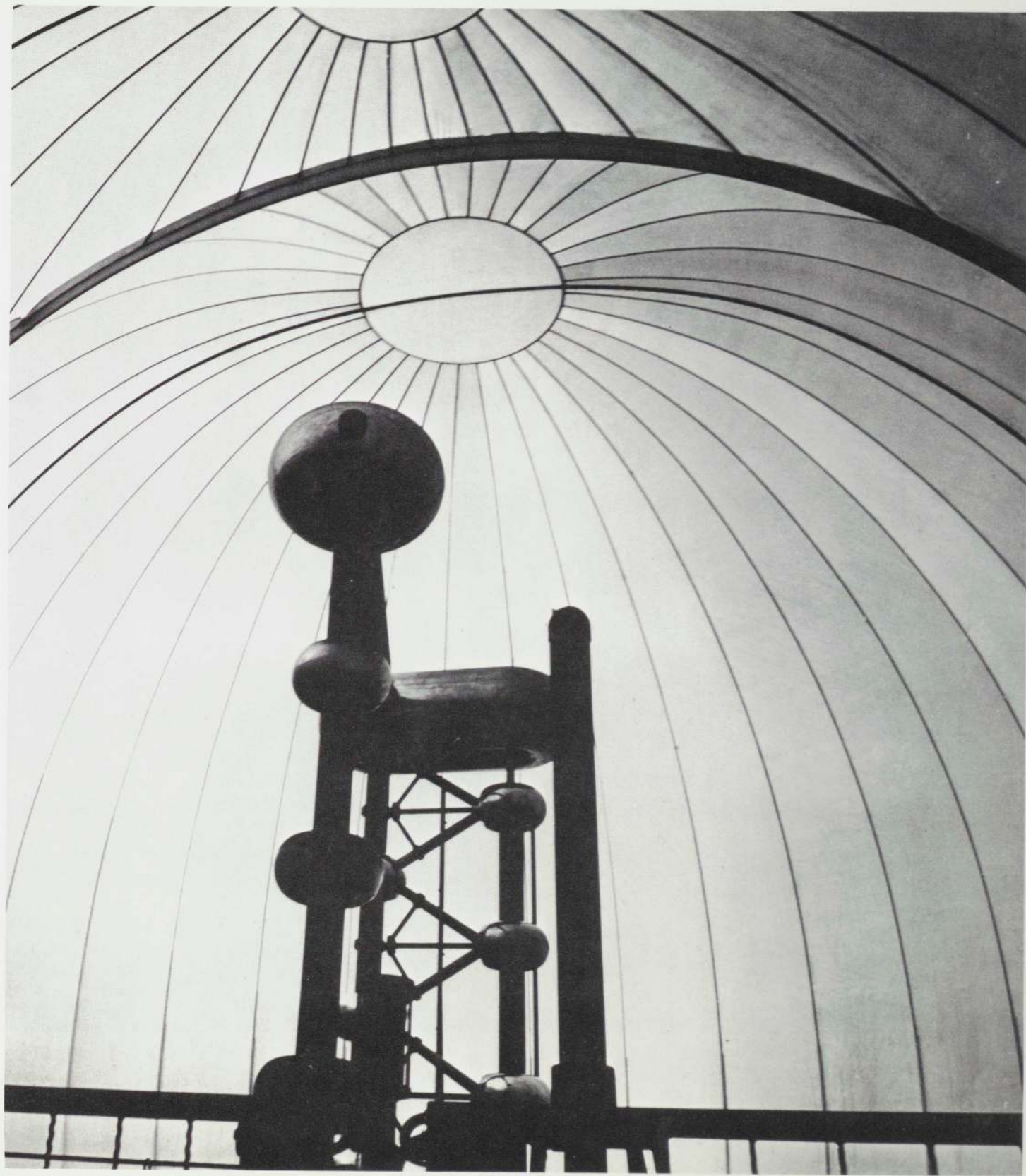
High-Voltage Test Laboratory, Cologne, 1966
