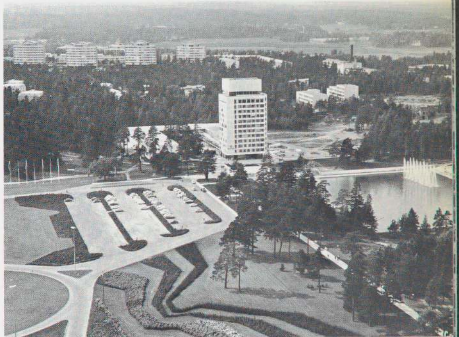
Tapiola Garden City, 6 miles from Helsinki, Finland. Developed since 1953 by the Finnish Housing Association, a private non-profit group, the town will house 17,000 with a lively interweaving of income levels, family sizes, and building types. The town center will serve over 100,000. Designed by Aarne Ervi and shown here, it is in the initial stages of construction.
