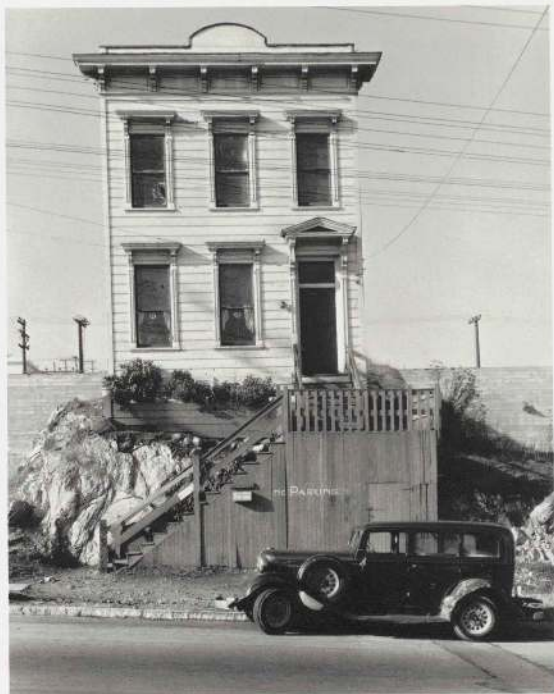
33. Tennessee Street, San Francisco December 28, 1949 (49-645)
