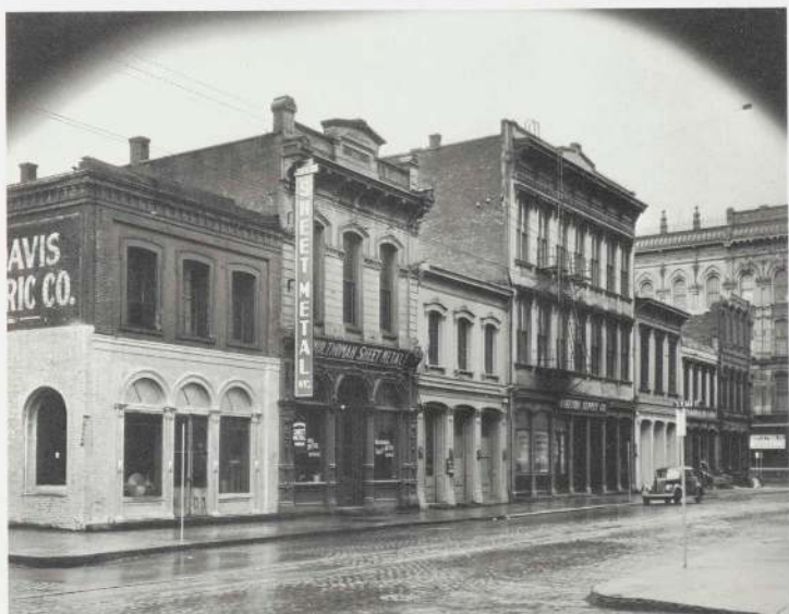
3. S.W. Front Avenue, Portland 1939 (39-53)
