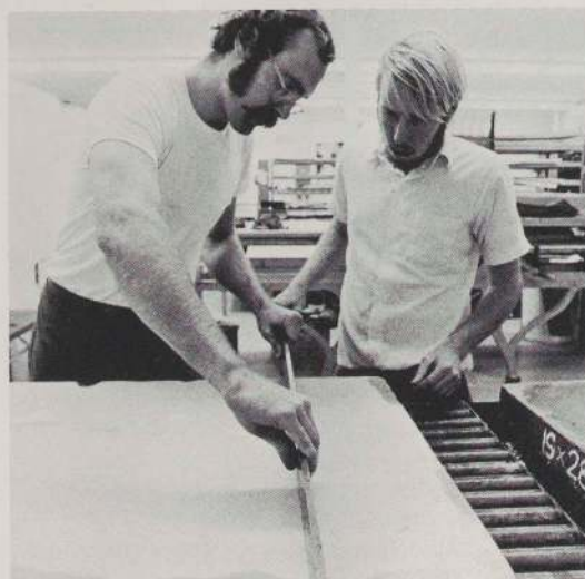
Stuart Henderson and Ron McPherson, printers, checking level of stone with a straight-edge Gemini, 1969
