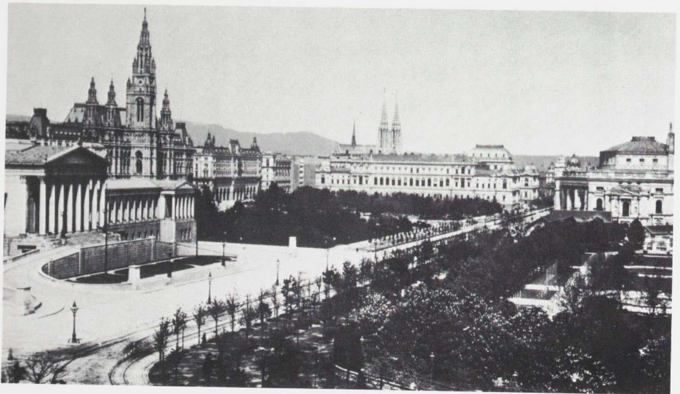
View of the Ringstrasse. c. 1888. From left: Parliament, Rathaus (City Hall), University of Vienna, and Burgtheater.
