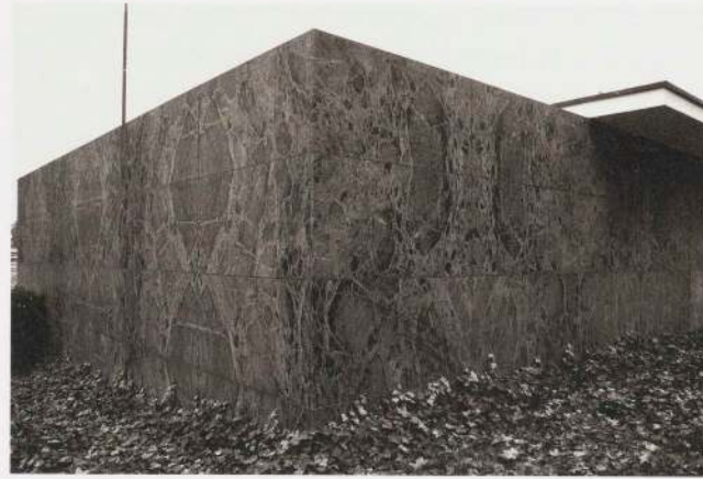
38. Ludwig Mies van der Rohe. German Pavilion, International Exposition, Barcelona. 1928–29. View of rear or garden facade and corner of the reconstruction of 1986. Photograph: Kay Fingerle, 2000
