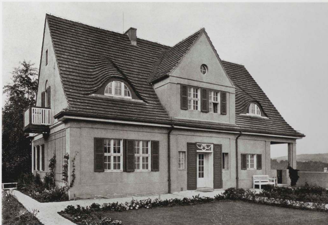
2. View of entrance facade, c. 1907
