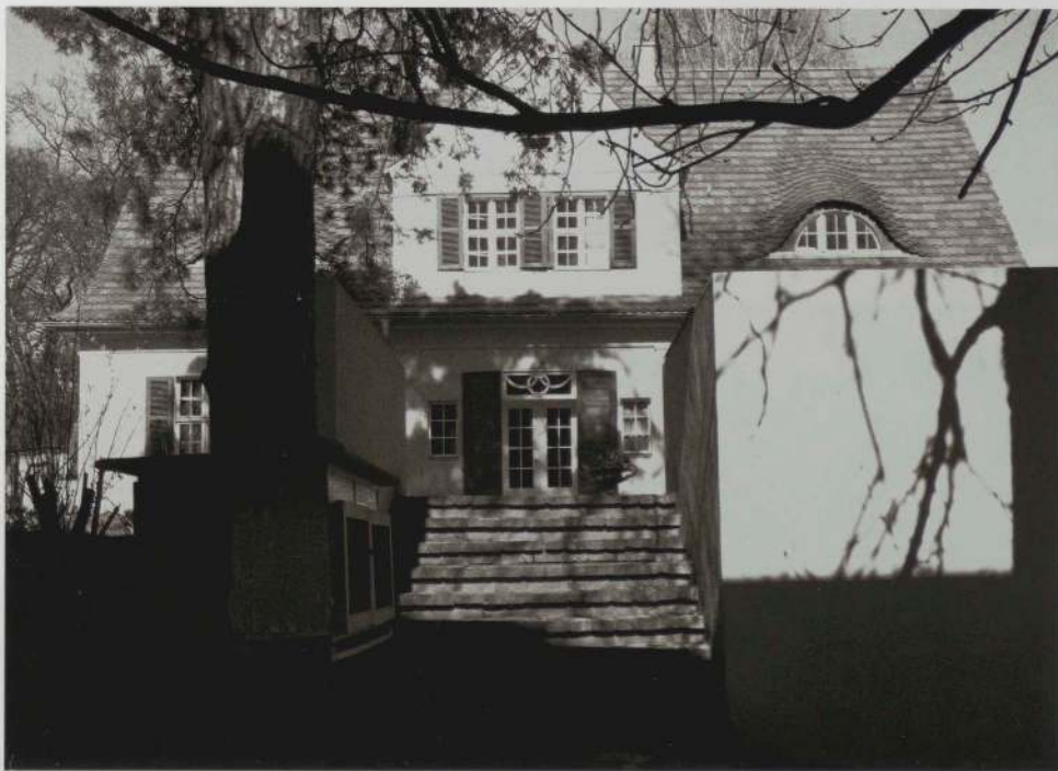
3. View of entrance facade from beyond garden stairs. Gelatin silver photograph, 11 \frac{1}{16} x 17 \frac{1}{16} " (50 x 45 cm). Photograph: Kay Fingerle, 1999
