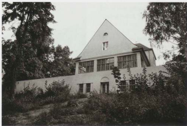
8. View of service area, rear facade. Gelatin silver photograph, 11 13/16 x 17 11/16" (30 x 45 cm). Photograph: Kay Fingerle, 1999
