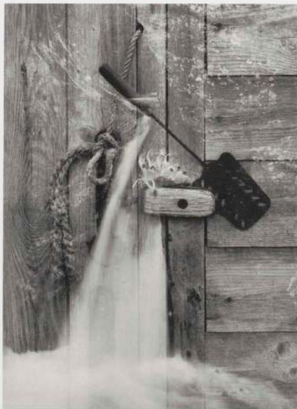
87. Vicinity of Lincoln, Vermont, with Texas Falls, Vermont Late October 1970 (70-16)
