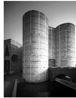
IMAGE THIRTY-ONE: Exterior Prayer Hall, Sher-e-Bangla Nagar, Dhaka, Bangladesh. National Assembly Building, 2002. Photograph: Raymond Meier
