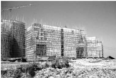
IMAGE THIRTY-THREE: Construction photo, National Assembly Building, Sher-e-Bangla Nagar, Dhaka, Bangladesh, c. 1970. Louis I. Kahn Collection, University of Pennsylvania, and the Pennsylvania Historical and Museum Commission
